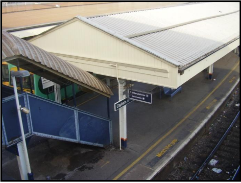
Canopy & Stairs that were removed.
